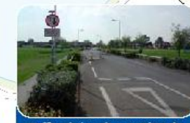
Traffic calming schemes reduce the speed of motor traffic and this one also provides cyclists with a fast, safe and comfortable route through.
