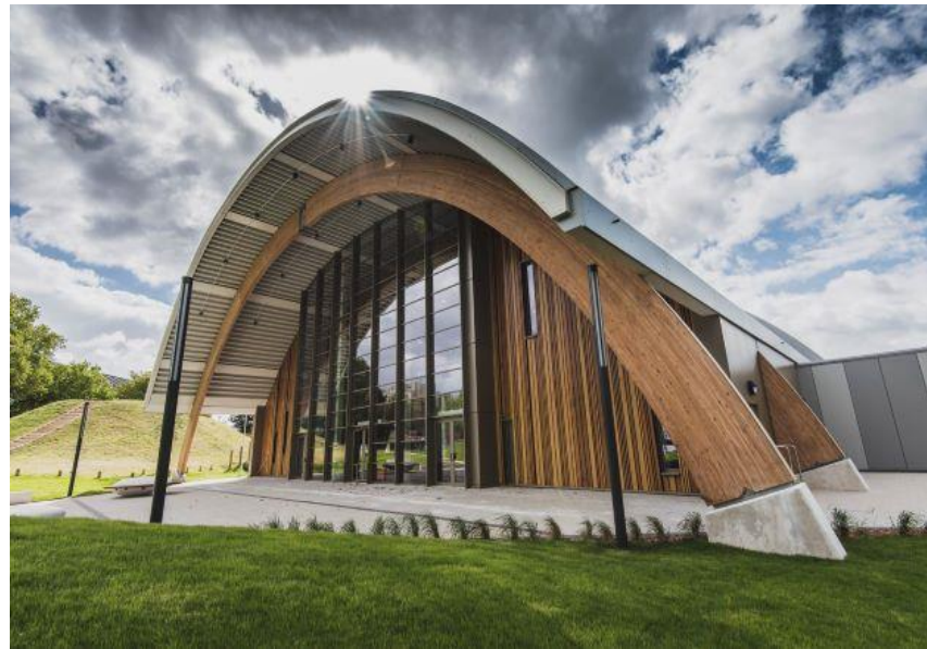
The Slough Ice Arena
