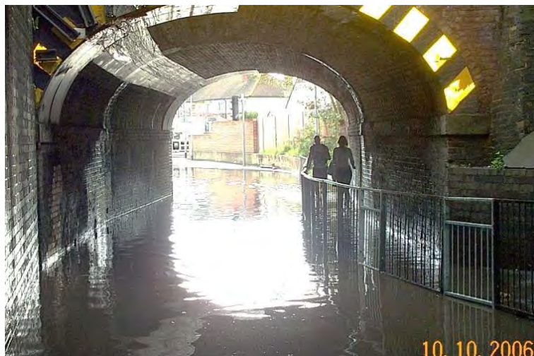
Figure 3-6: Flooding in Station Road, October 2006 (Refer to Figure 12 for photo location)
