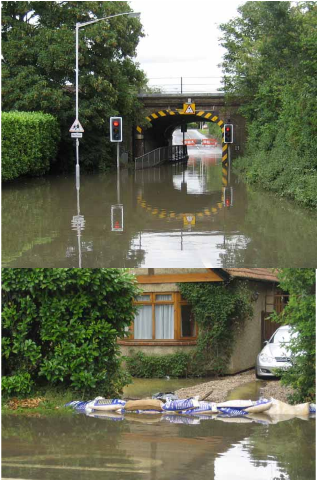
Plate B1 Flooding along Huntercombe Lane North at the railway bridge
