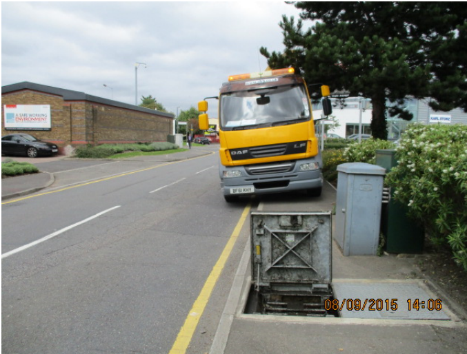
Figure 2-1 SBC visiting the Thames Water pump station
