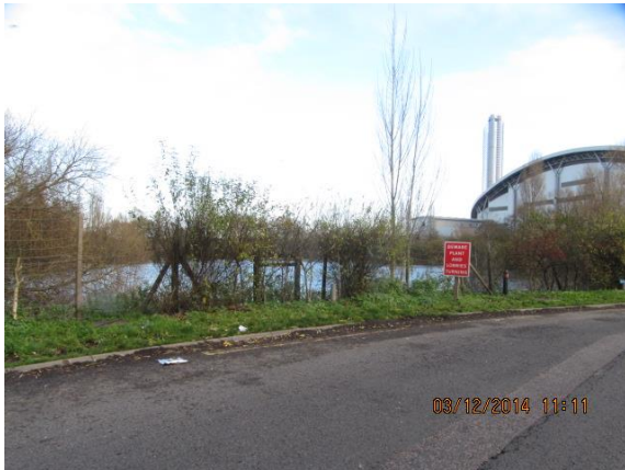
Colnbrook West Lake penstocks
