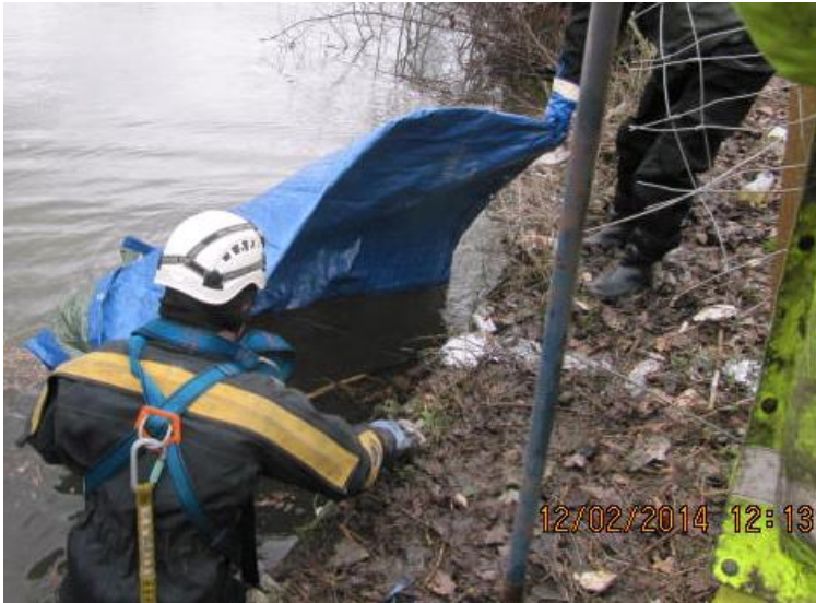
SBC sealing the main penstock at Colnbrook West Lake.
