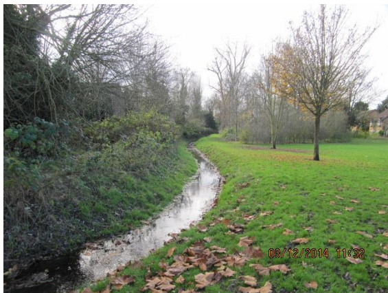
Upgraded drainage channel
