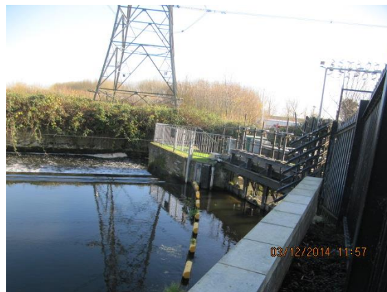
Horton Mill Weir and assets
