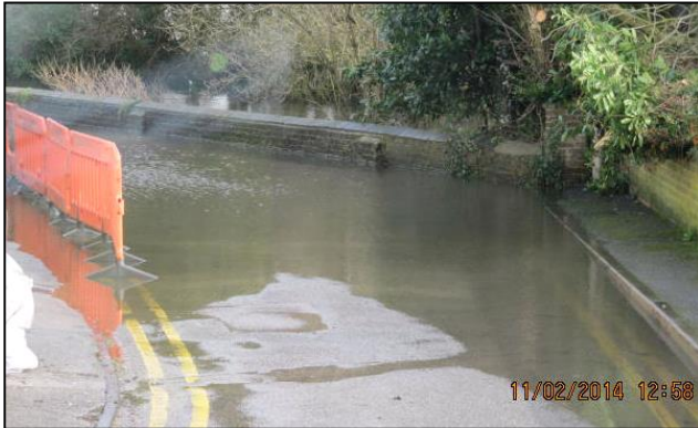
Flooding on Mill Street
