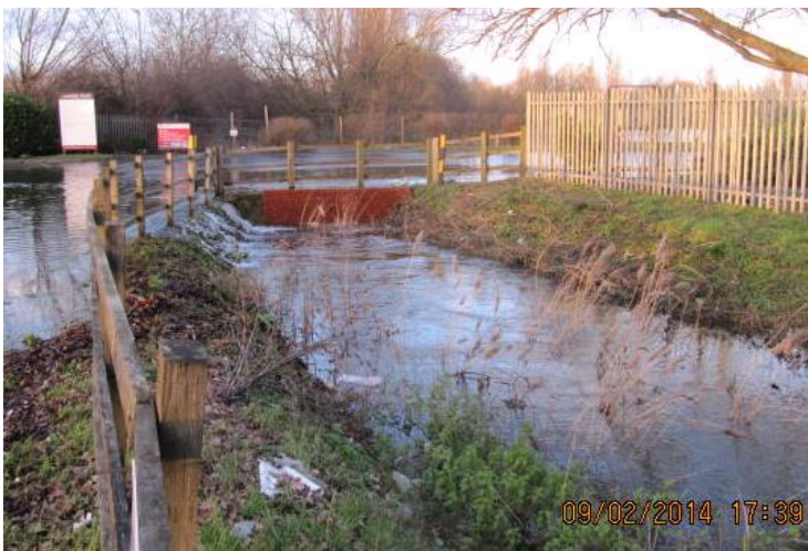
Water from West Lakes overtopping Lakeside road and draining into Hawthorn Ditch
