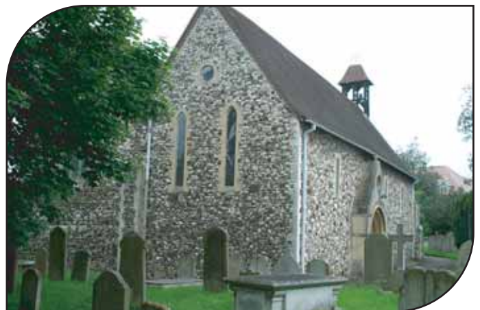
St Laurence's Church from South East
