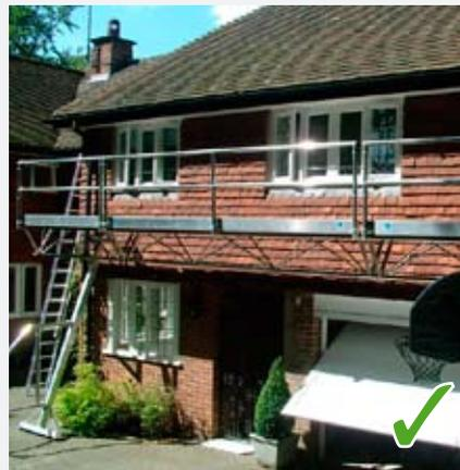
◀ This photograph shows a properly erected proprietary working platform. Such system scaffolds should be erected in accordance with the suppliers instructions.
