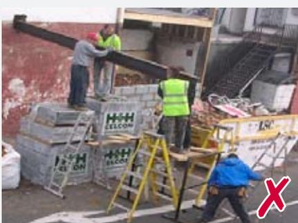
◀ These workmen are lifting and installing a steel beam by hand from unsafe working 'platforms' located in a live roadway.
