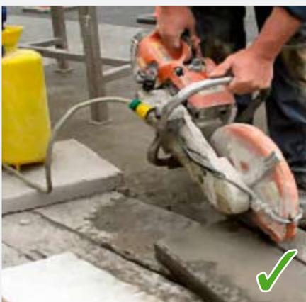
▲ Water suppression is being used here to properly control the dust. Water is fed from the yellow container direct to the cutter area.
