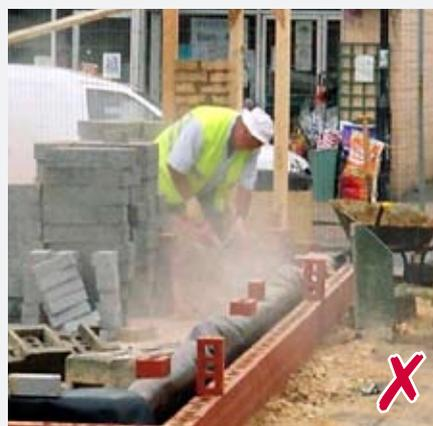
▲ No measures are being taken to control the dust generated by the use of this disc cutter. Workmen and others will be inhaling the damaging dusts.
