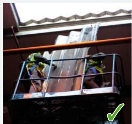
This shows a mobile elevating work platform being used to replace a rooflight from below the roof. ▶
