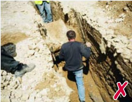
◀ The workman in this trench is at significant risk of being killed should the sides of the excavation collapse. No-one should ever enter an unsupported excavation.
