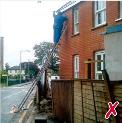
◀ Gutters are being fixed from an unsecured ladder placed in the road at an unsafe angle. The work being done makes it impossible for the user to hold the ladder.
