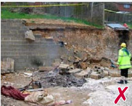
◀ A workman died when this wall fell during remedial work on the wall.
