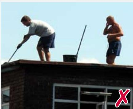
◀ Repairs to flat roofs (including single storey) present a significant risk of falling and injury. These men are refelting a flat roof without suitable edge protection.
