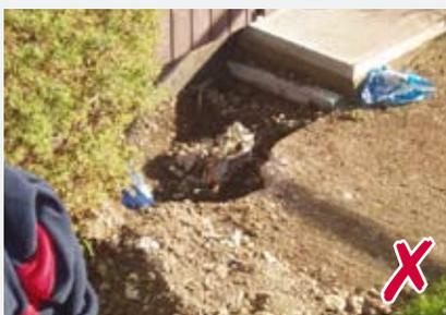
Underground cables are commonly struck ► during ground work. This can cause explosions, flash burns and electrocutions. Obtaining drawings from utility companies is not enough. Cable locating devices should be used with drawings and safe digging techniques to avoid excavating over the top of an indicated line of a cable.
