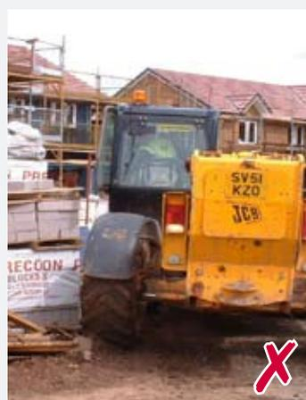
◀ This shows a very poorly organised site. The forklift truck is manoeuvring in a very restricted area where other workers may be present and materials are stored. No effective steps have been taken to separate vehicles and pedestrians.
