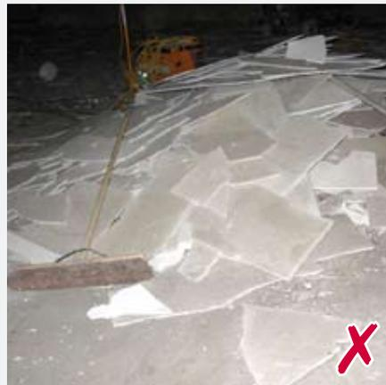
▲ This shows what can happen when a survey is not undertaken or the findings not acted upon. Asbestos insulating board is shown strewn on the floor having been swept with a broom.
