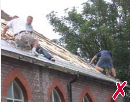
◀ These men are re-roofing a sloping roof without edge protection to prevent falls. This is highly dangerous.
