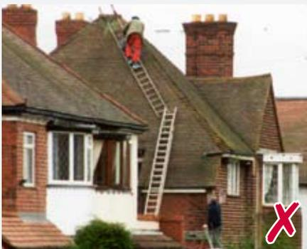
◀ Roof ladders can be used to make minor repairs to sloping roofs. The ladders must be suitable and properly used. This photograph shows ladders being used in a manner that could easily lead to a catastrophic fall of the ladders and the roofer from the slope.
